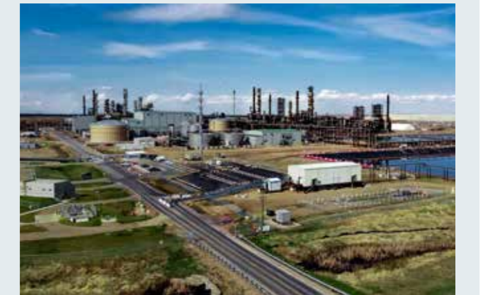
Sturgeon Refinery Aerial. 写真提供：Alberta Carbon Trunk Line
