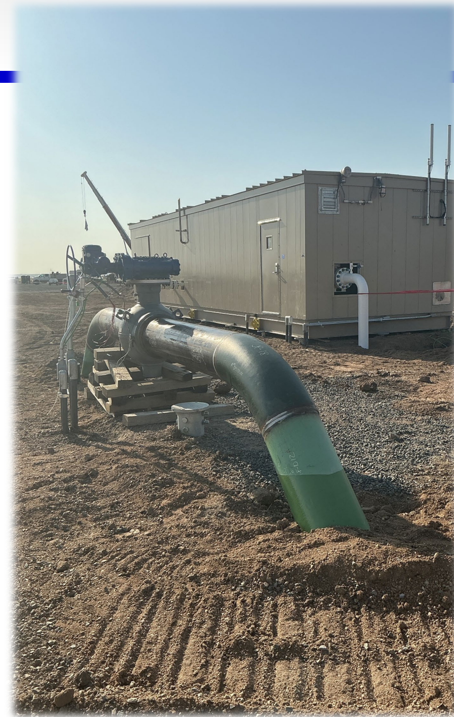
Tallgrass High Plains Carbon Storage, LLC Juniper I-1 wellhead and flowline/metering building prior to initial commissioning injection test, 6/28/2025, photos by TH
